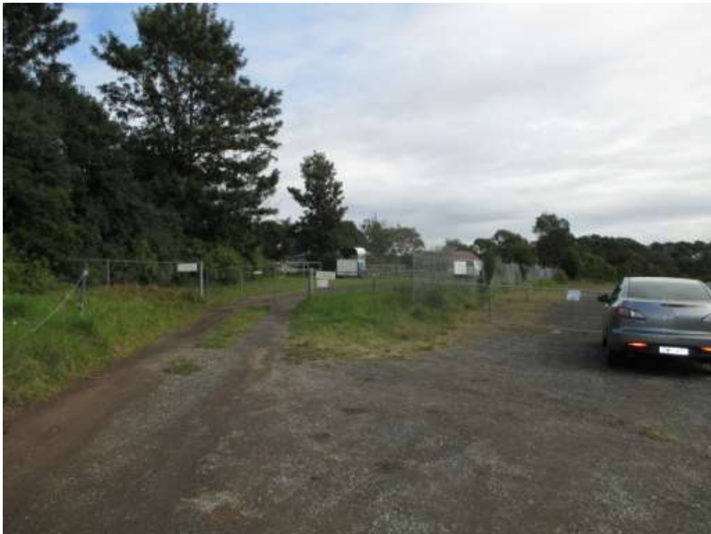
Figure 4: View of site from Epping Road looking south-west (RMS reservation on the right side of photo)
